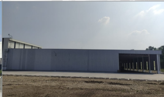
EXPAND FACTORY REAR VIEW
