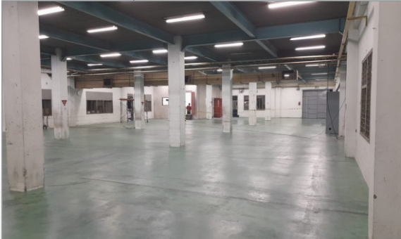
CONCRETE AREA PRODUCTION
