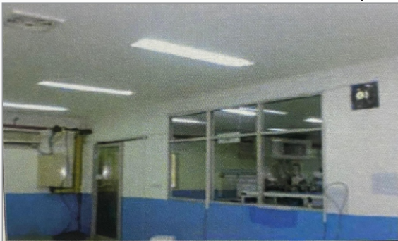
INSTALLATION OF PARTISION OFFICE
