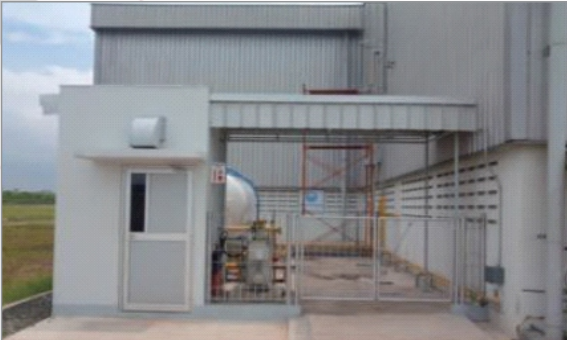
BUILD GAS ROOM
