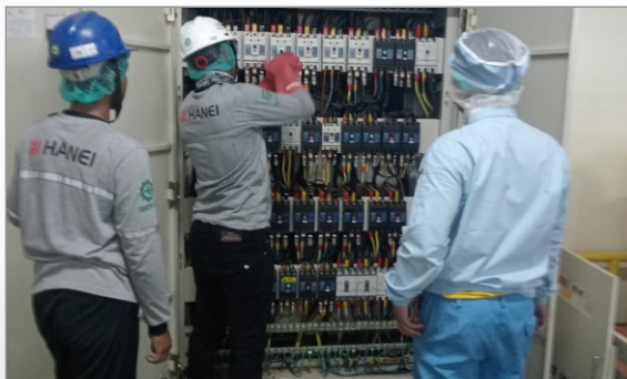
POWER CABLE LIGHTING TO PANEL EXISTING
