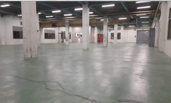
CONCRETE AREA PRODUCTION
