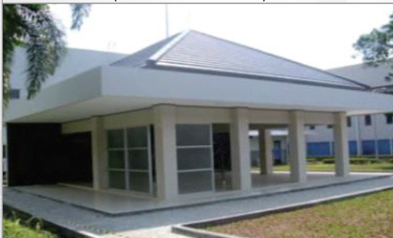
MUSHOLLA RENOVATION : 216 m2
