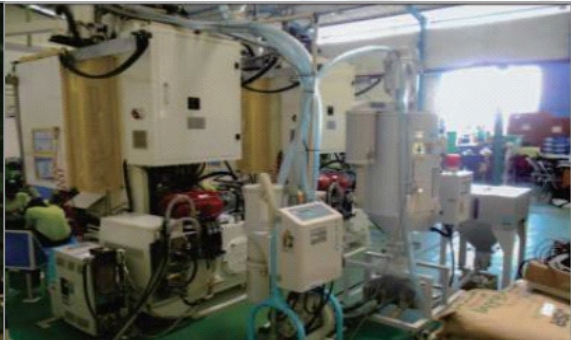
RUBBER EXTRUDER MACHINE INSTALLATION
