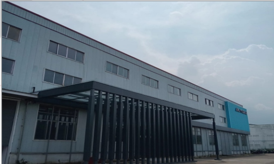
BUILD CANOPY IN AREA LOBBY
