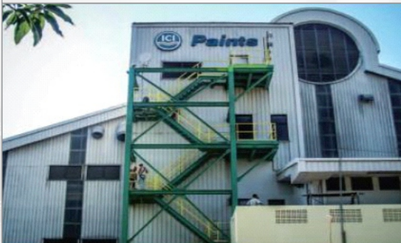
PAINTING ALL BUILDING
