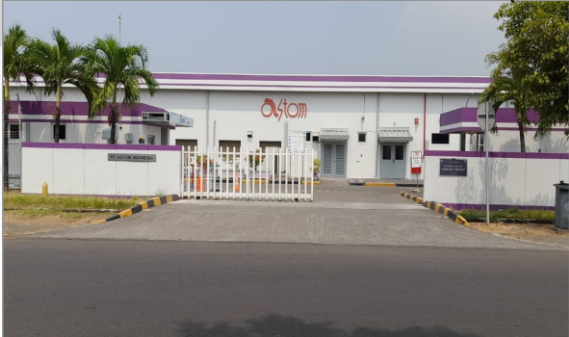
REPAINTING ALL BUILDING
