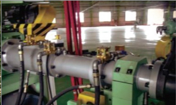
RUBBER MOULDING MACHINE INSTALLATION
