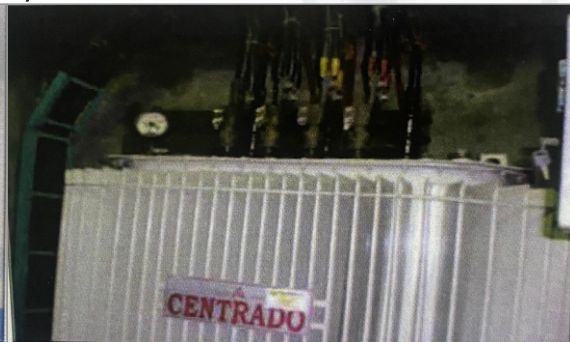
INSTALLATION OF TRANSFORMATOR 2000 KVA
