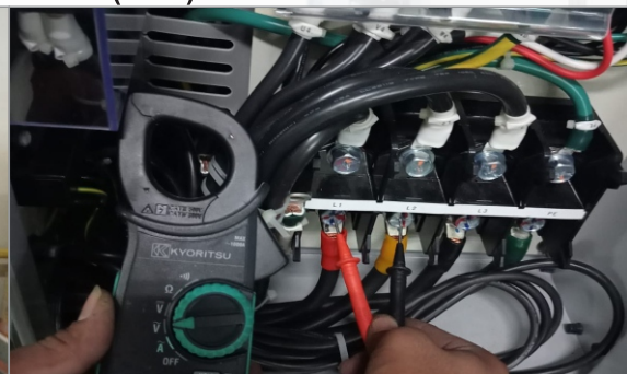
TESTCOM AND TEST VOLTAGE
