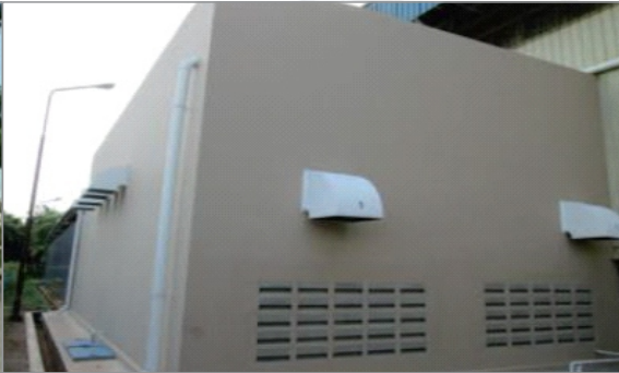
COMPRESSOR ROOM : 82 m2
