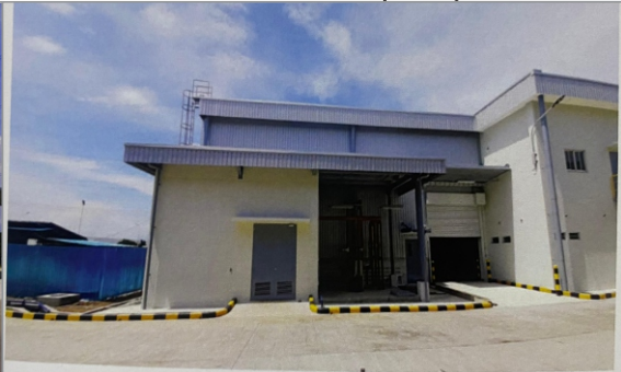
NEW PUMP ROOM
