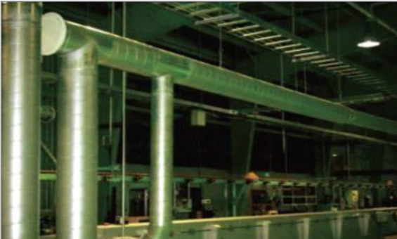
INSTALLATION EXHAUST DUCTING
