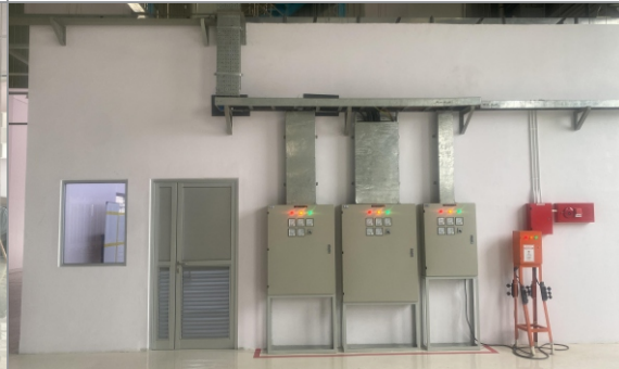
INSTALLATION PANEL AND BUILD MAINTENANCE ROOM
