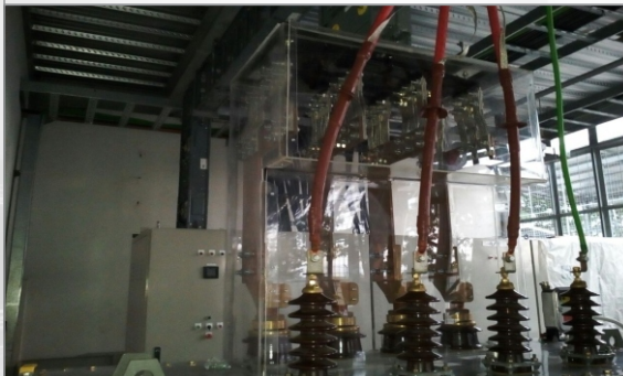
INSTALLATION TRAF0 2500 KVA
