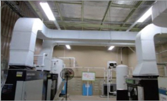
INSTALLATION COMPRESSOR & EXHAUST DUCTING
