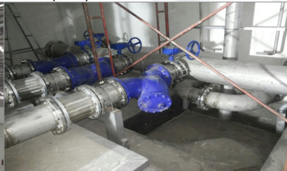
INSTALLATION PIPING WATER SUPPLY
