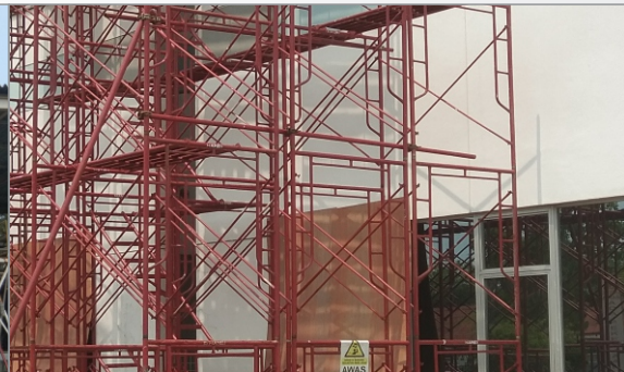
REPAIR WALL CRACK
