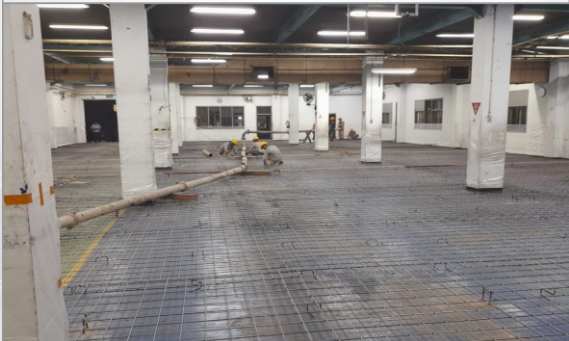
CONCRETE AREA PRODUCTION
