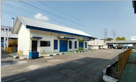
EXPANSION ELECTRICAL ROOM
