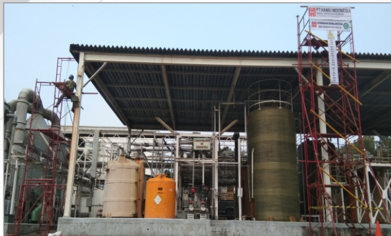
REPAIR ROOF CHEMICAL AREA
