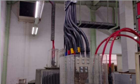
INSTALLATION CABLE TRAF0 2000 KVA
