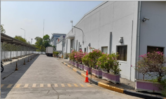
REPAINT ALLUMINIUM GLASS
