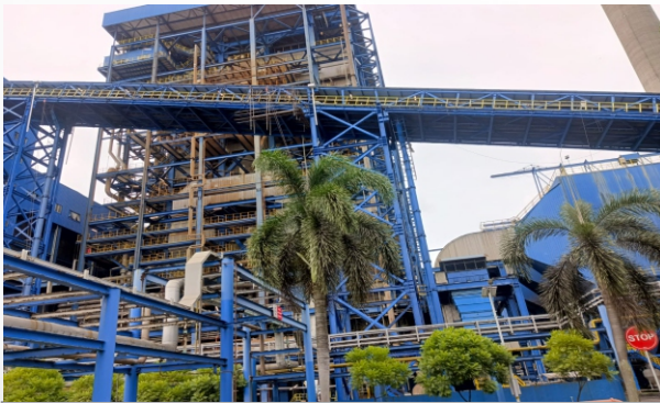
INSTALLING ADDITIONAL STRUCTURE CONVEYOR
