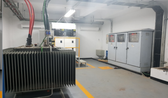
INSTALLATION OF TRANSFORMATOR
