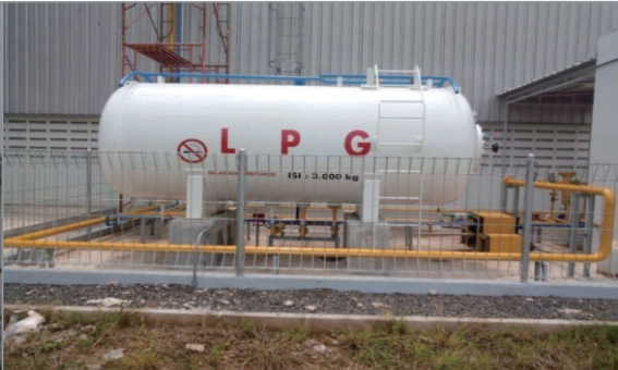
LPG 3 TON TANK INSTALLATION
