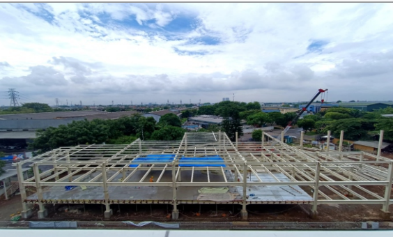
ERECTION STEEL STRUCTURE ( AIR VIEW )
