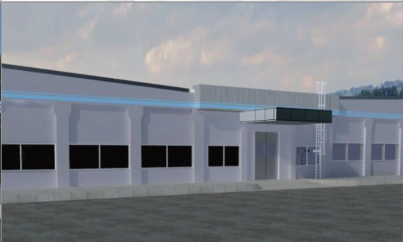
SWITCH STORE : 920 m2
