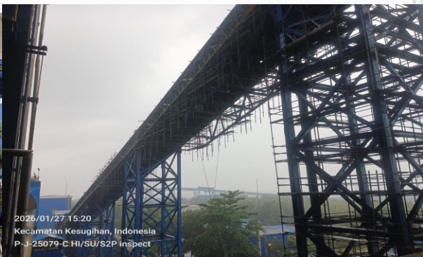
DISMENTLING CREMONA CONVEYOR
