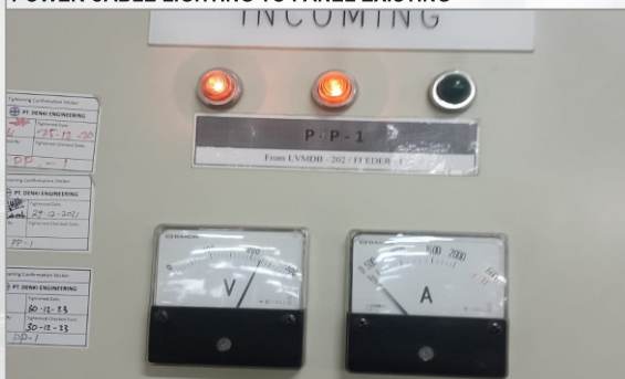
INSTALLATION NEW PANEL
