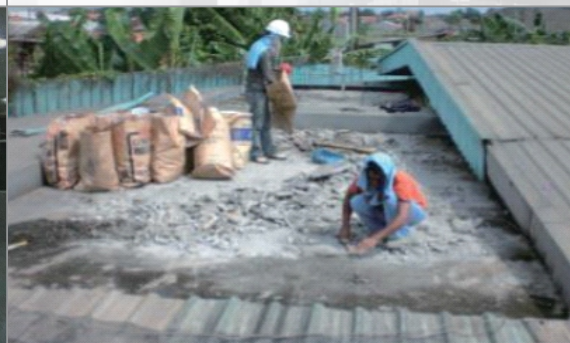
REPAIR ROOF CONCREATE
