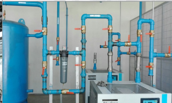
INSTALLATION PIPING AIR COMPRESSOR
