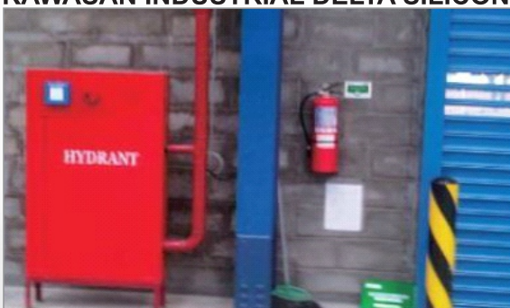
HYDRANT BOX INSTALLATION
