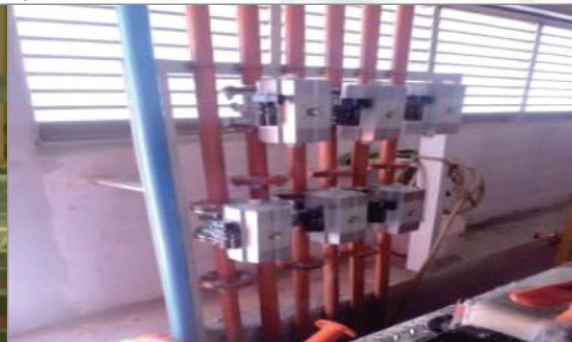
INSTALLATION AUTOMATIC VALVE
